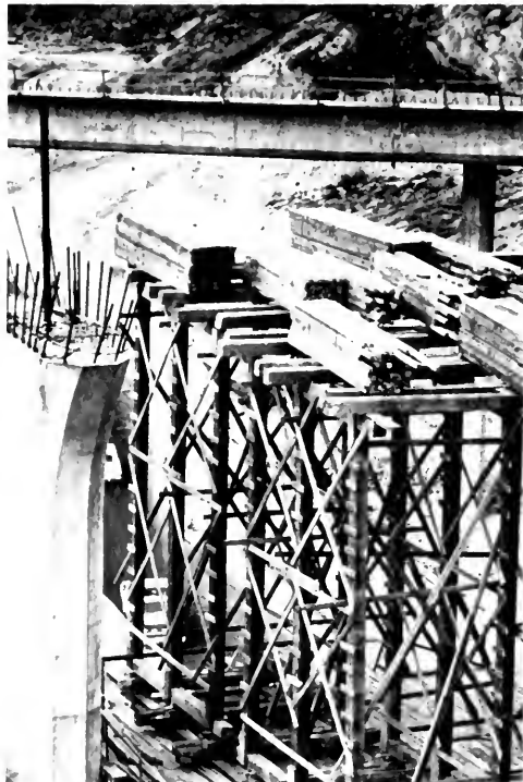
Photo 21. Timber falsework at the Golden State Freeway and State Highway 14 interchange.
